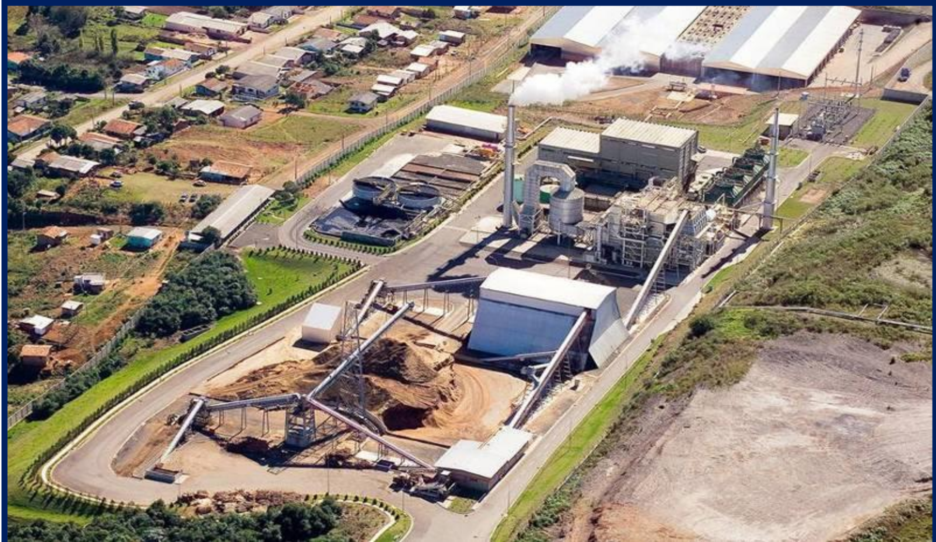
CENTRAL TERMICA BIOMASA RENOVBABLE
